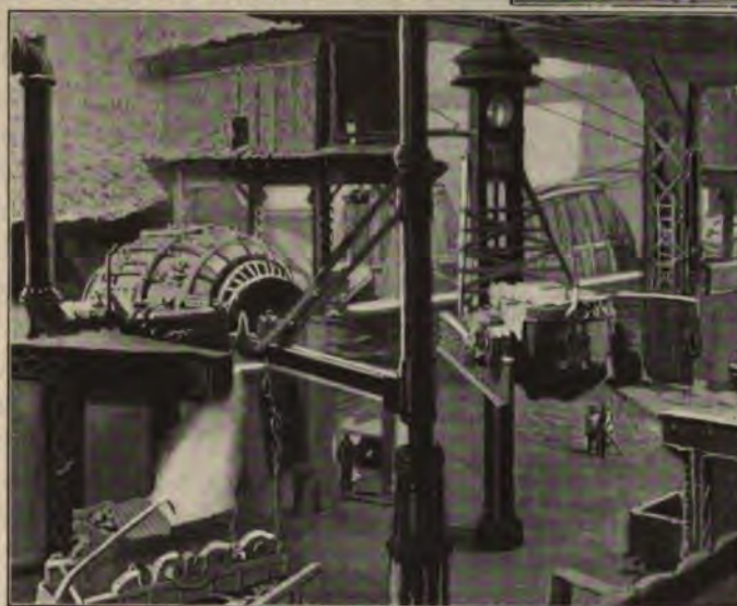
Making steel near Pittsburg. The iron is melted in the furnace, poured into little cars called ladles, rolled to the mixer where it is treated, and then poured into the converter. This cut shows a converter ready to be loaded with melted iron from the mixer near by in the center. When it is loaded the converter is turned so that it stands as the other two converters. Hot air is forced through the melted iron, which raises it to white heat, burning out all the impurities and converting it into steel. During this process out of the mouth of the converter pour flames, burning gases and millions of sparks.
